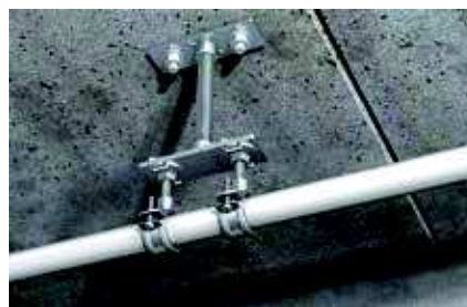
Plastic pipe with fixpoint installation
